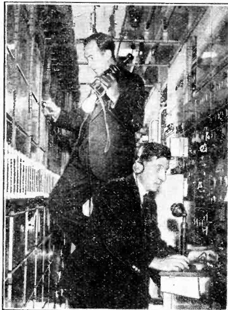
BEHIND THE SCENES. B.B.C. engineers checking amplifier performance behind one of the panels in the Control Room at Broadcasting House.
